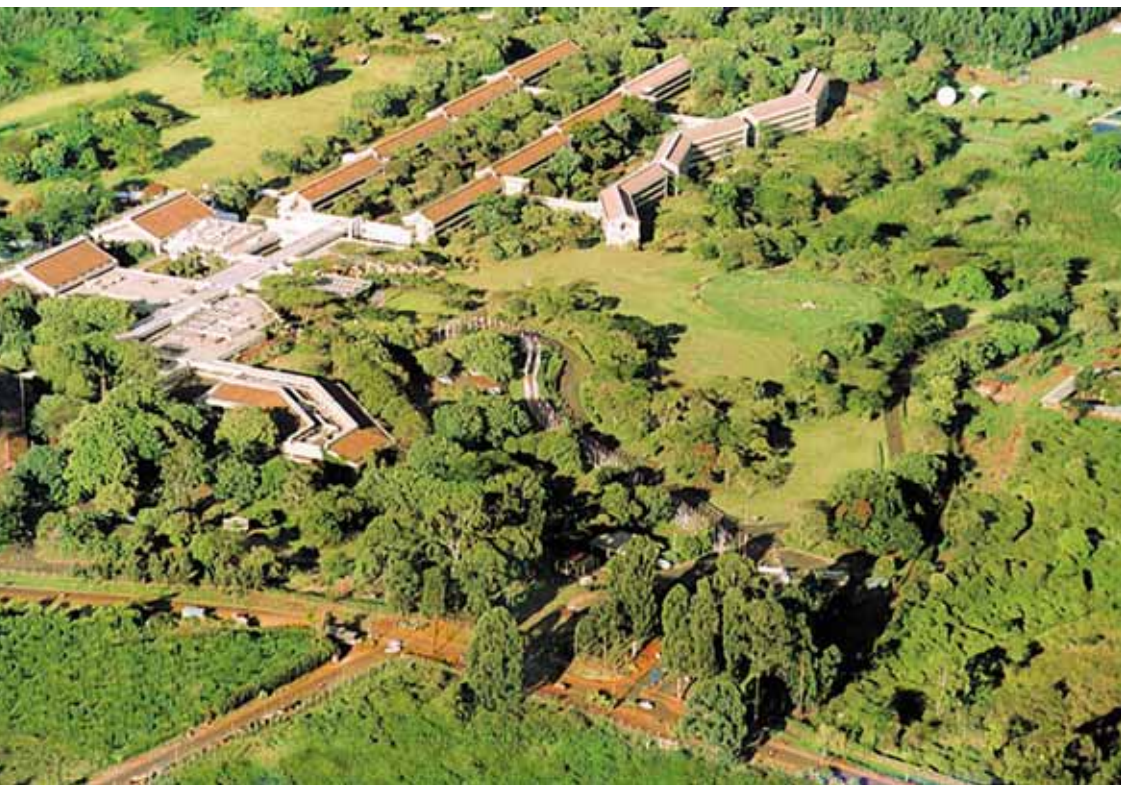
Aerial view of the UN Complex in Gigiri, Nairobi.
